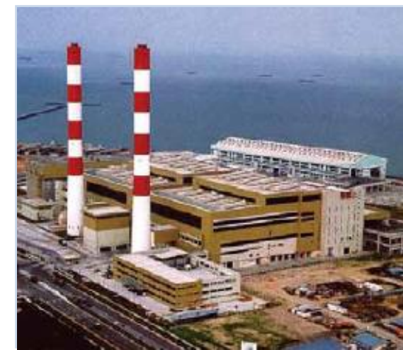
WtE plant in Beijing, with capacity to handle 1,600t/day, by Takuma Co., Ltd.
