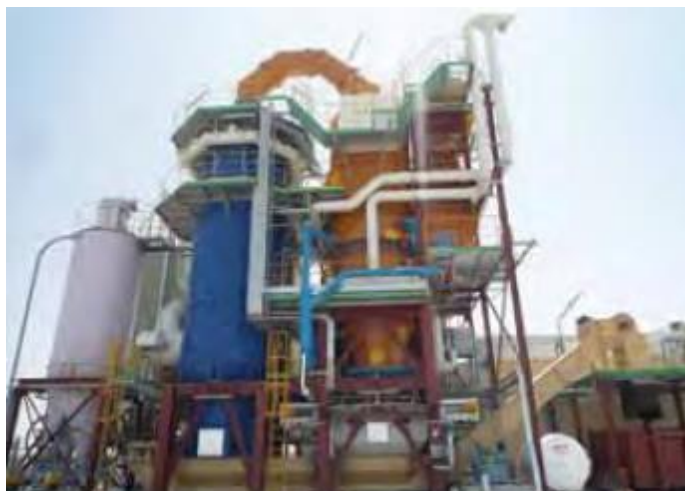
The medical waste incineration facility in Dubai
