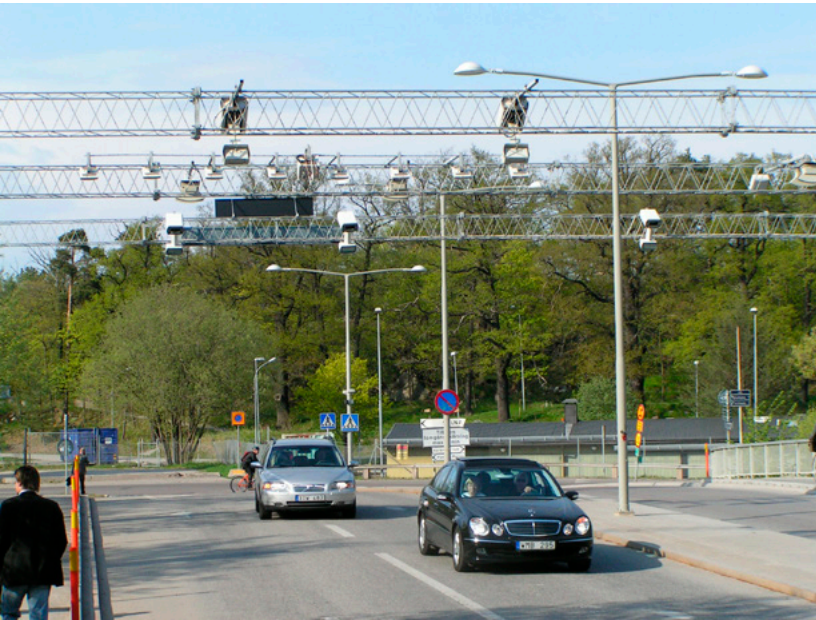
Figure 56: Congestion charge check points deliver useful data for planning and policy evaluation, Stockholm. © Manfred Breithaupt, 2006
