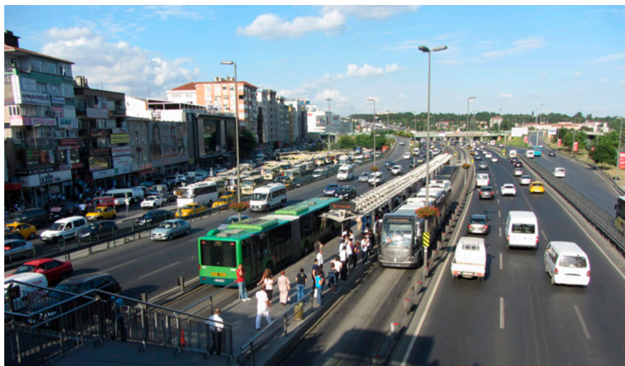
Figure 2a: The BRT system in Istanbul ensures free passenger flow even at times of heavy congestion.
