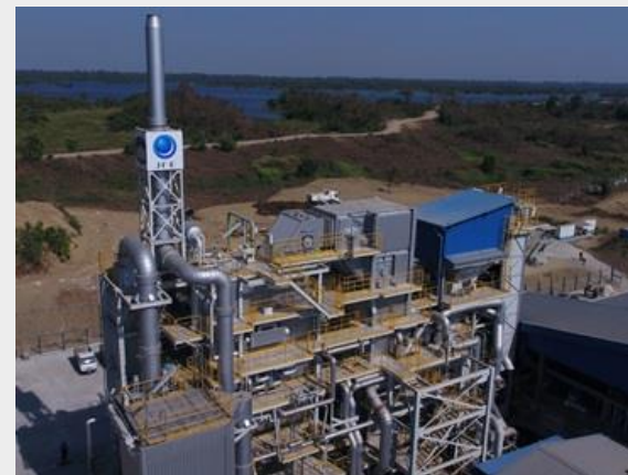
WtE plant completed in April 2017 in Yangon
