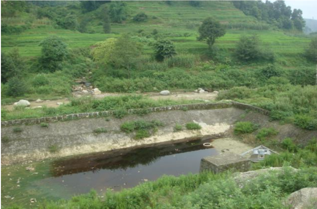
Leachate Treatment Pond
