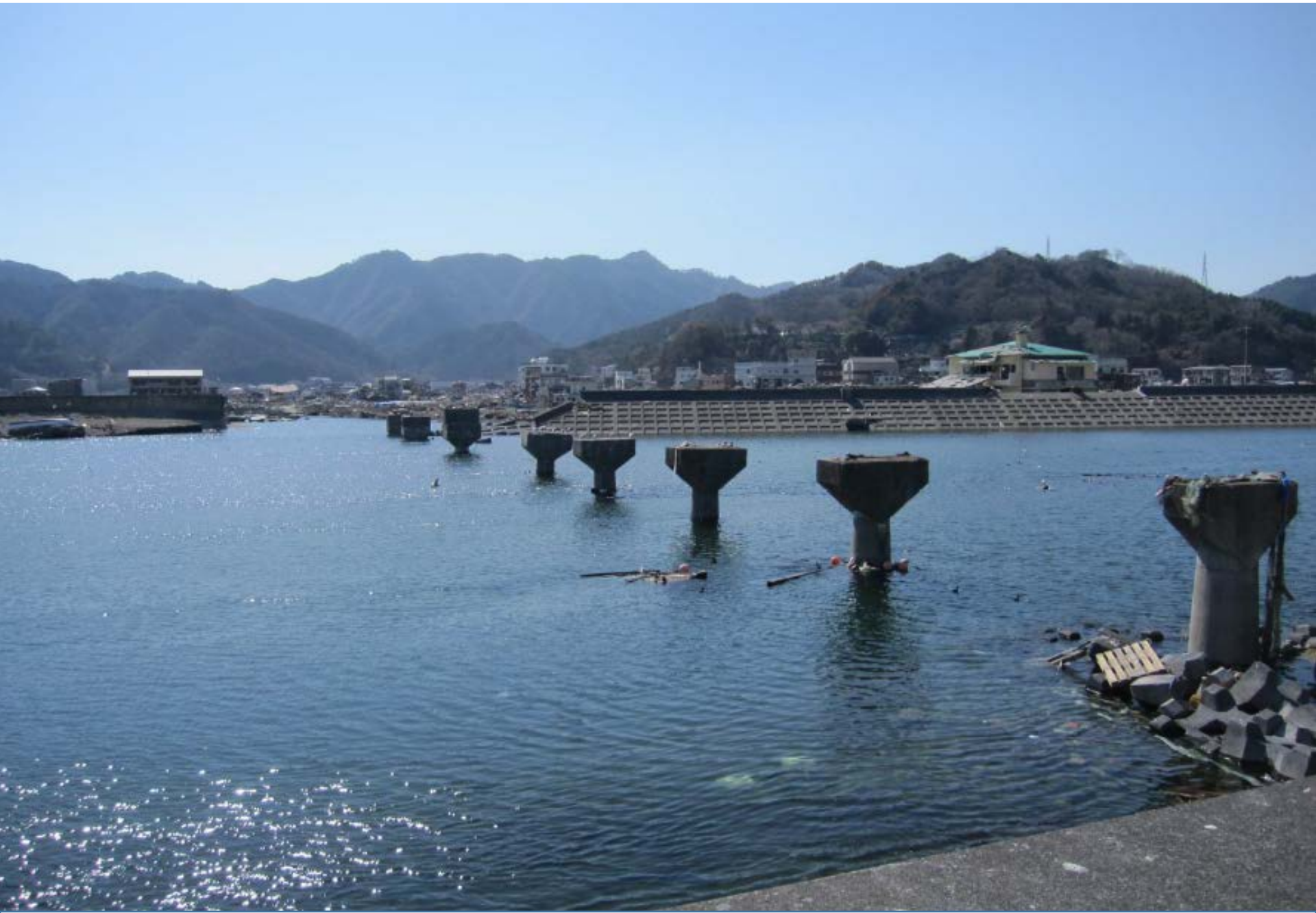
At Great East Japan Disaster in 2011, Rail road was washed away
