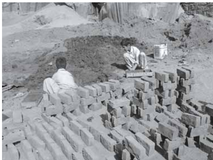
Application of a PRA method encourages a community to participate in analyzing and identifying their vulnerability to disaster
