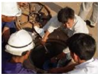
Water supply project at Phnom Penh
