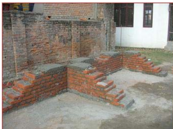
Load Bearing Wall
