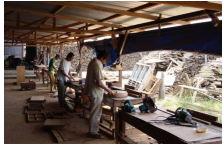
Reparation of window frames and doors
