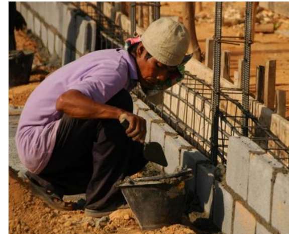
Construction activities after the tsunami
