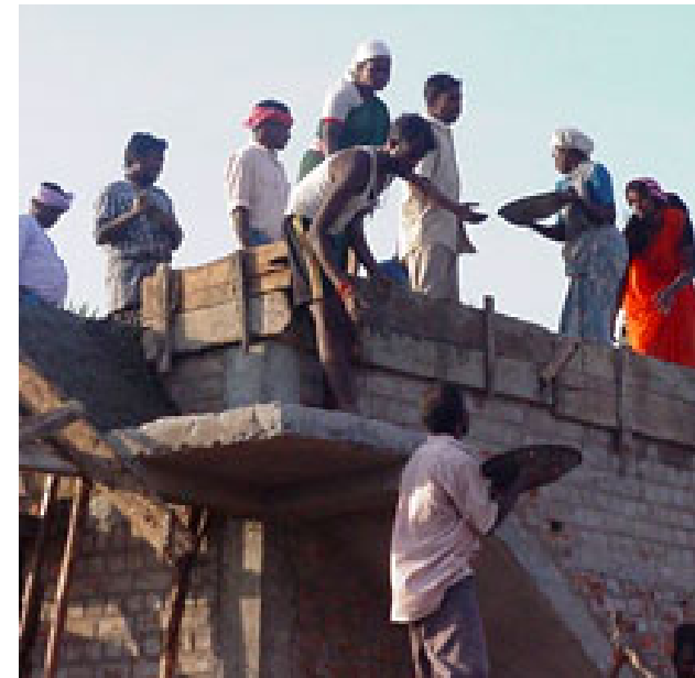
Construction activities after the tsunami
