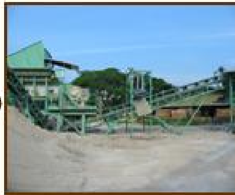
2) Preliminary crushing and removal of ferrous metals
