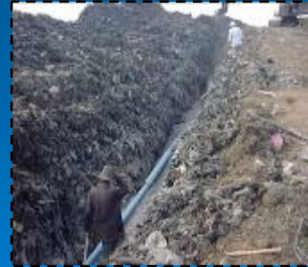
Biogas from landfill at Rachadeva (950 kW)
