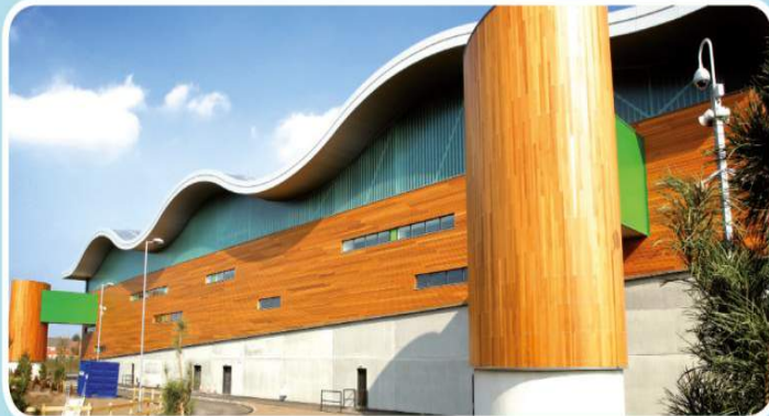
Gillmoss Materials Recovery Facility
