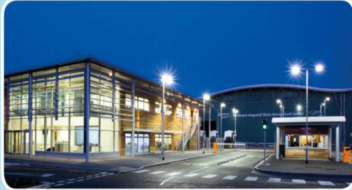
Southwark Integrated Waste Management Facility
