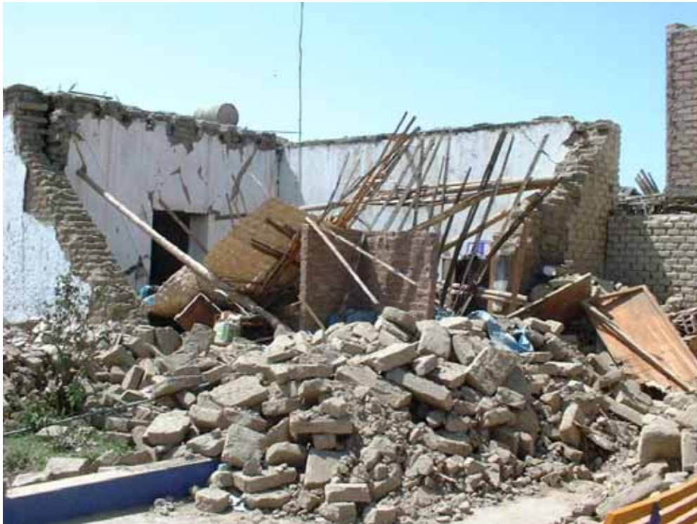
Photo 1: Destroyed adobe house in Ica City
