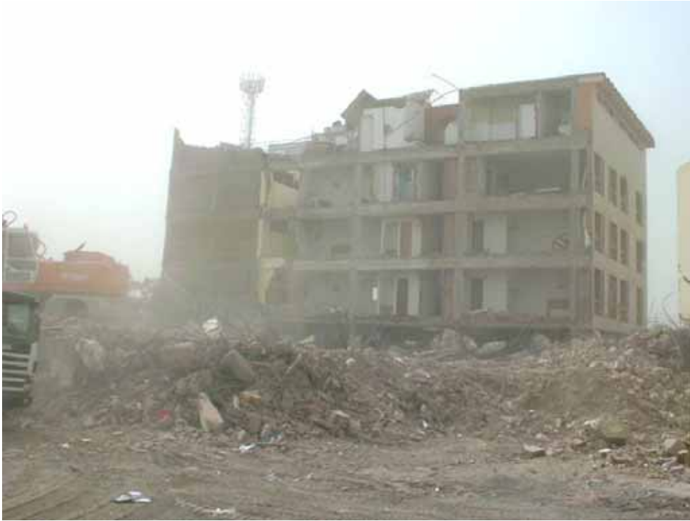
Photo 3: Demolition of five-story Hotel Embassy in Pisco City
