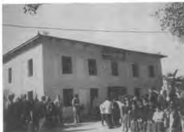
Retrofitted school in Kathmandu, Nepal
