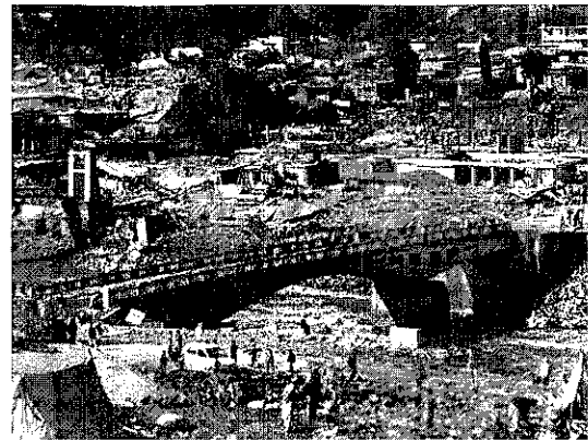
Photo2: Damaged Area in Balakot
