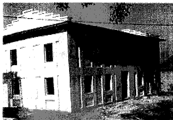
Photo3: School Earthquake Safety Initiatives Before and After Retrofitting
