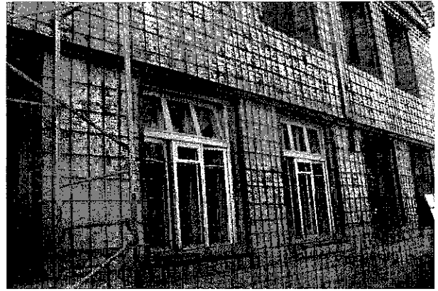
Reinforcement of masonry school building
