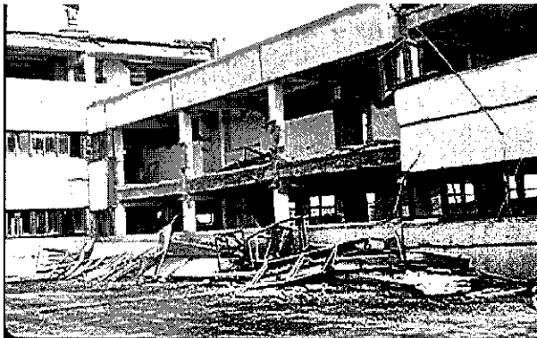
Damage of frame panel school building, Gazli 1984
