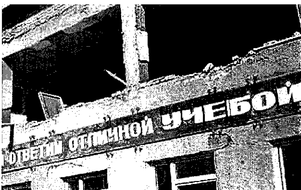
Damage of RC frame with brick filling school building, Gazli 1984
