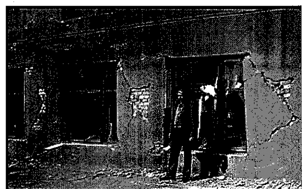
Damage of masonry school building, Gazli 1984
