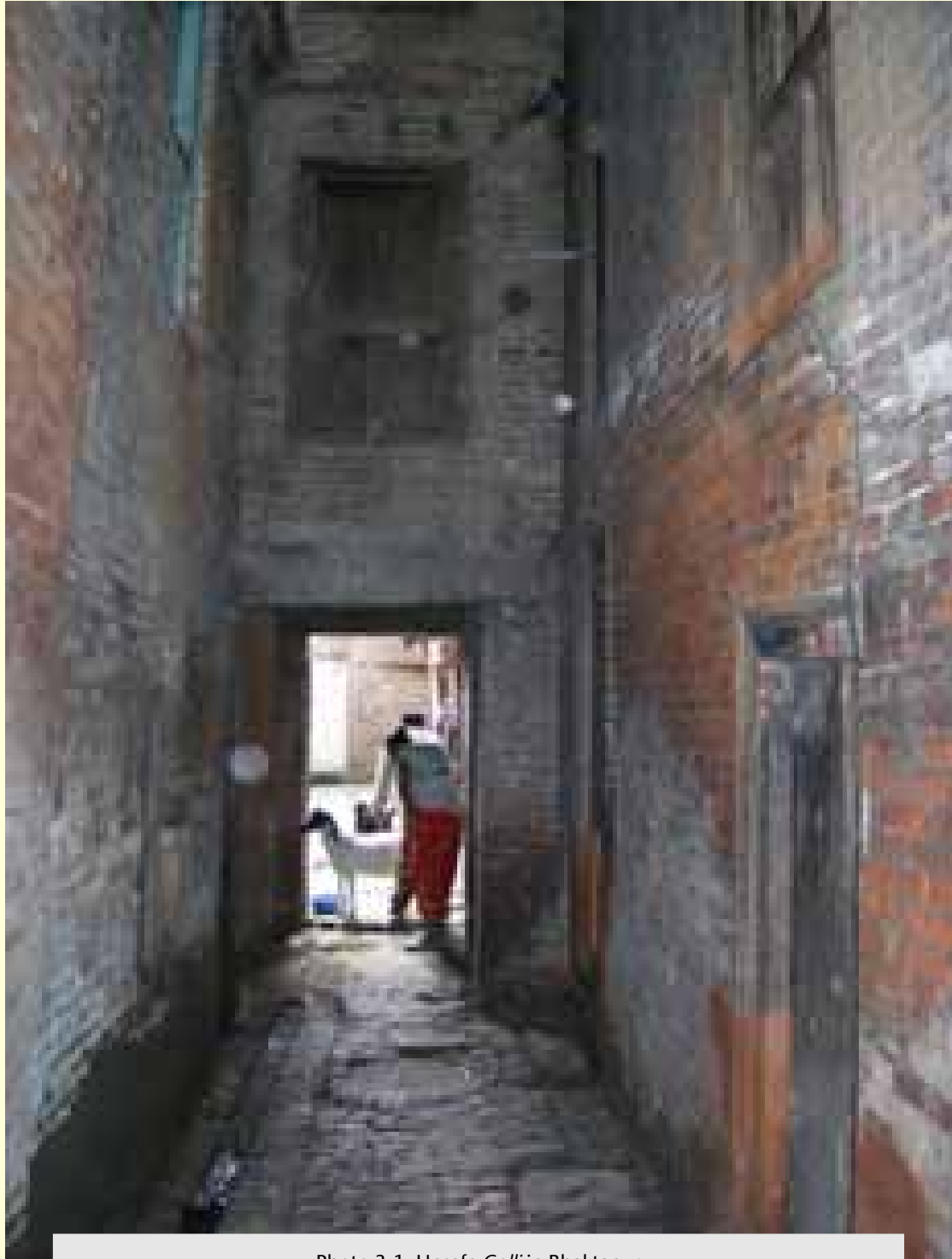
Photo 3-1: Unsafe Galli in Bhaktapur
