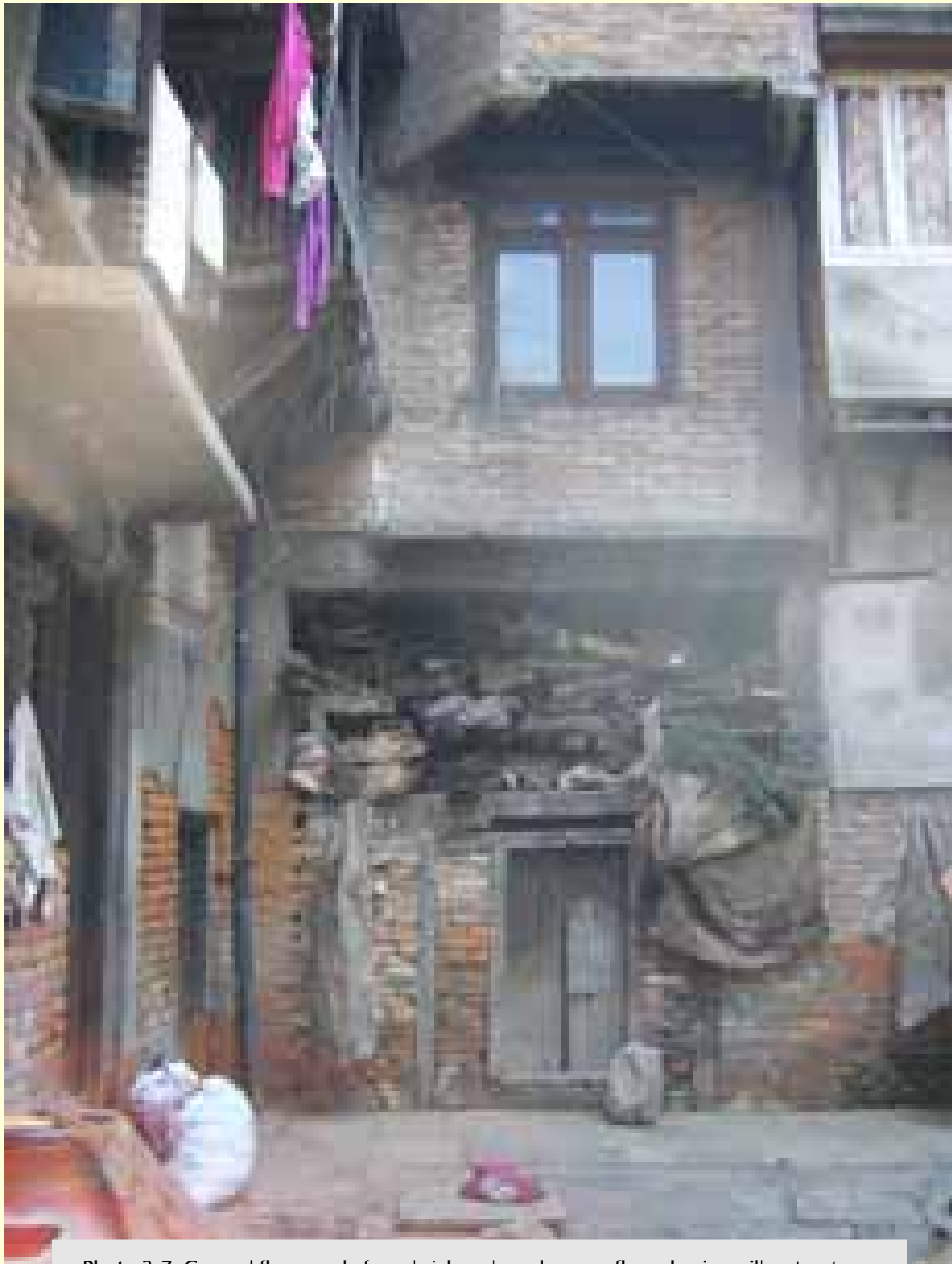
Photo 3-7: Ground floor made from brick and mud; upper floors having pillar structures
