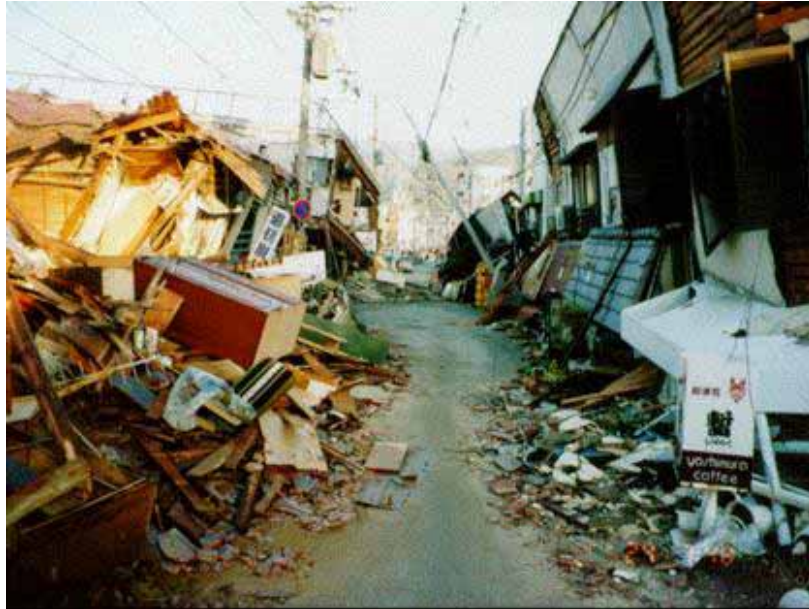
Photo 1: Collapsed old wooden houses
