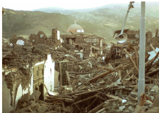
Photo 1: Damage to adobe constructions in the 1970 earthquake
