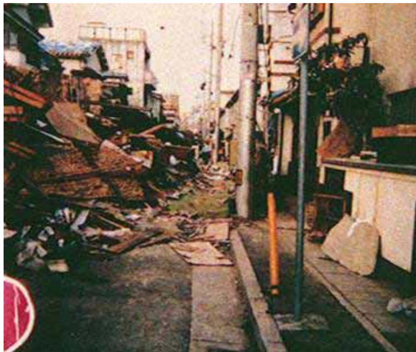
Photo 2: Road covered by collapsed houses
