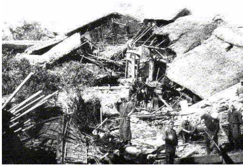
Photo 1: Damage of timber houses by the 1891 Nohbi Earthquake
