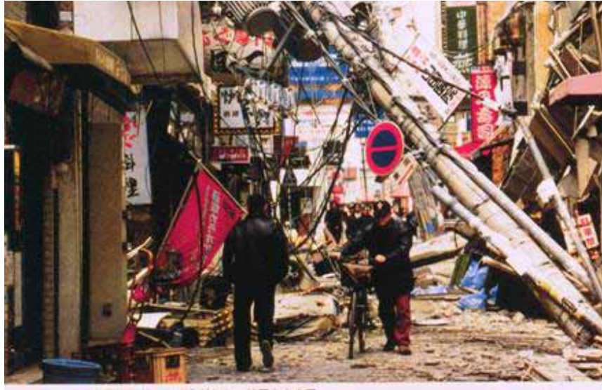
Photo 3: Collapsed electric light poles
