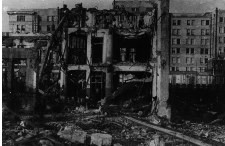
Photo 2: The Naigai Building near completion collapsed
