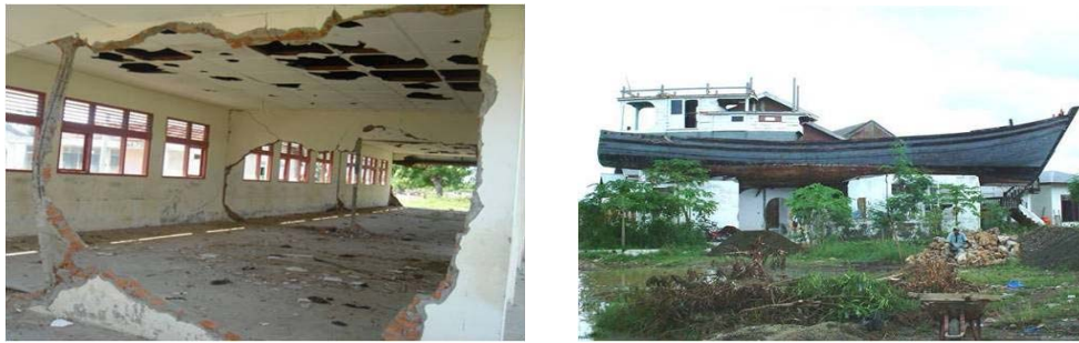
Figure 3. Damaged Masonry School (Left) and Remained Ship in the Residential Area (Right), Banda Aceh, Indonesia, December 2007
