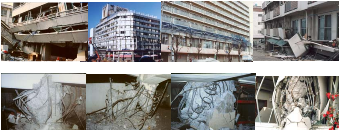
Figure 8. Reinforced concrete buildings in the 1995 Kobe disaster
