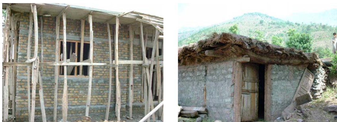
Figure 4. Reconstructed House (Left) and Traditional House in the Region (Right), Pakistan, March 2006
