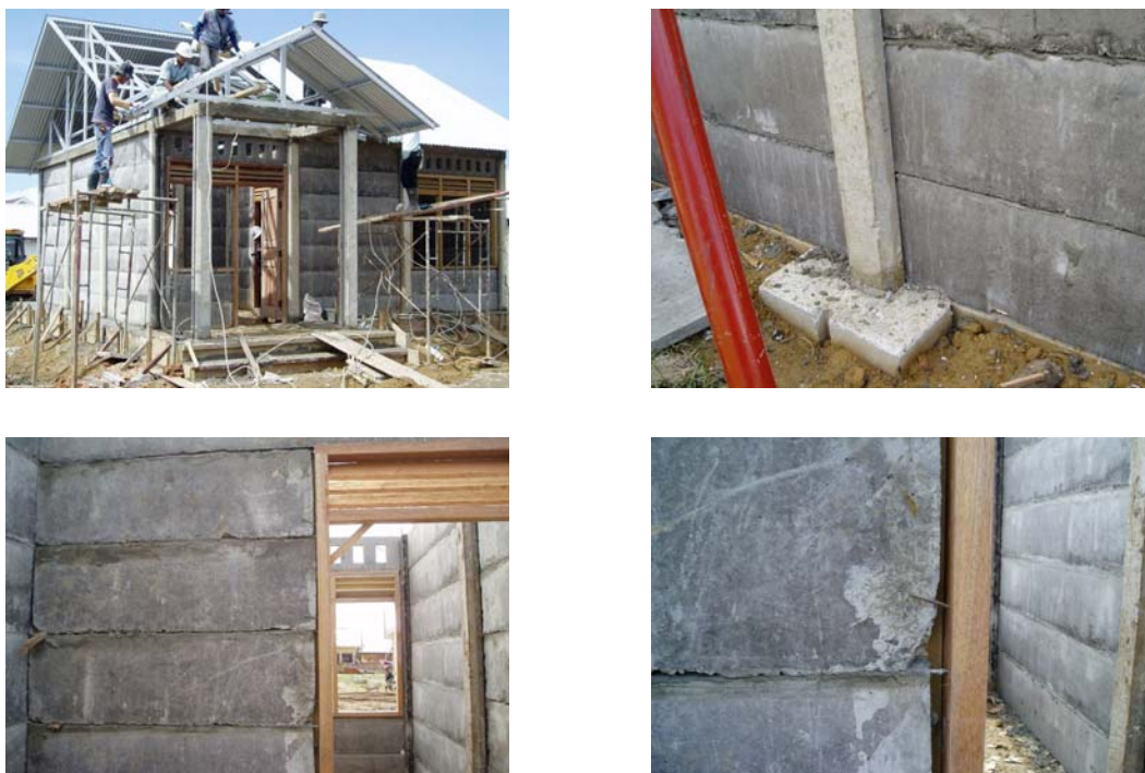
Figure 6. Walls using extra large size blocks with poor connections
