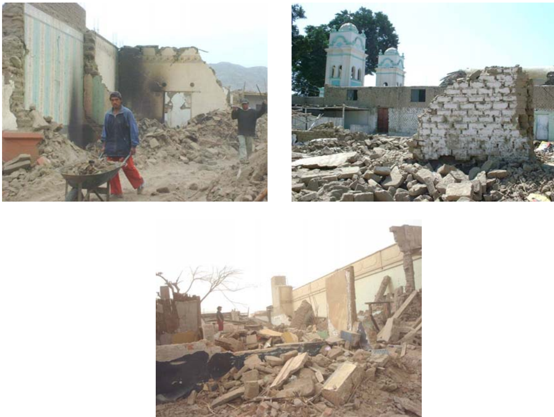
Figure 8. Recovery Works (Left), the Traditional Construction in Peru (Right), and the Damage caused by the Earthquake (Bottom), Pisco, Peru, August 2007
