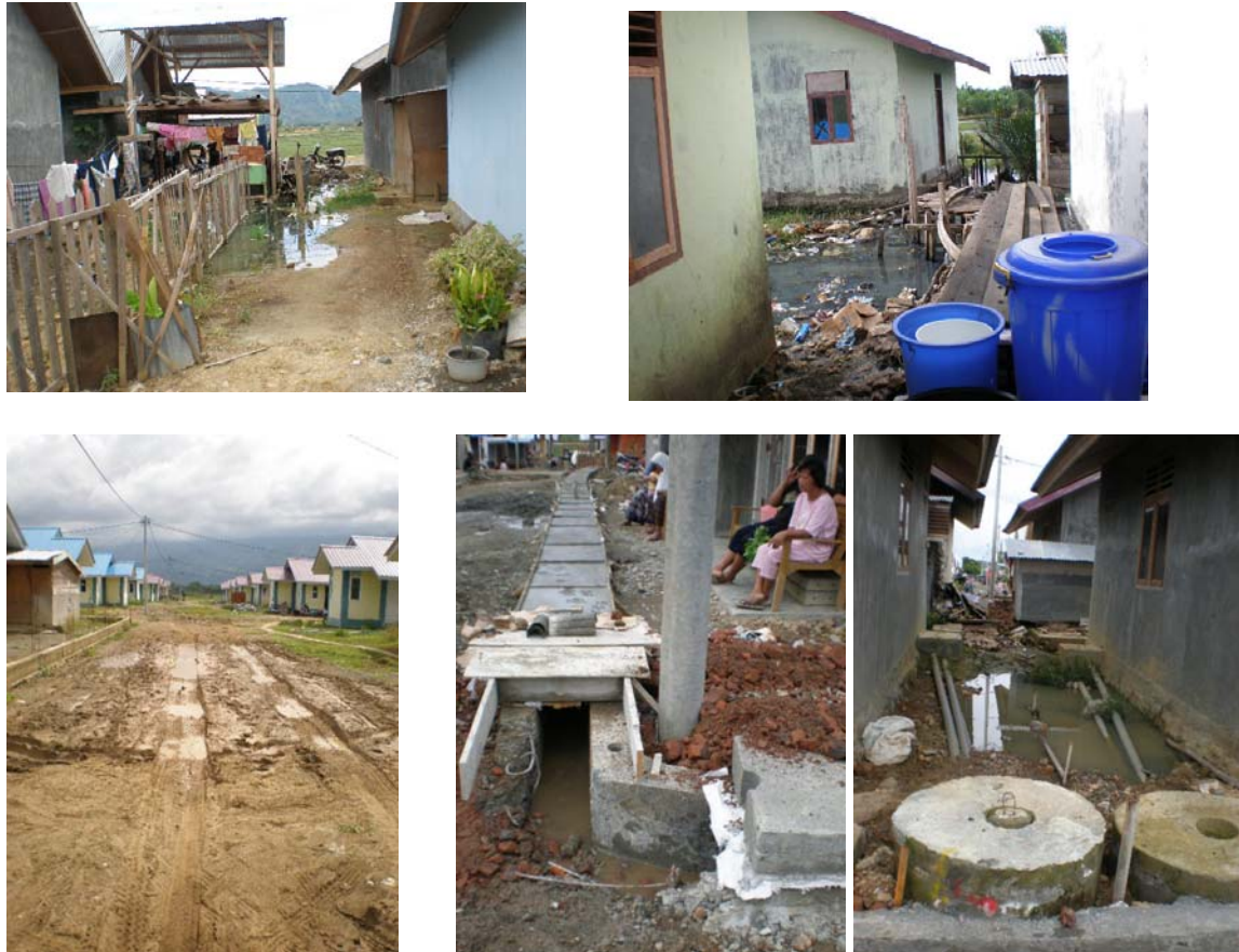
Figure 10. Site engineering construction activity did not run parallel with the site layout planning. All pictures were taken at the end of November 2008 (Aceh)
