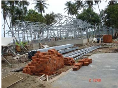
Figure 9. Light weight steel construction (Aceh)
