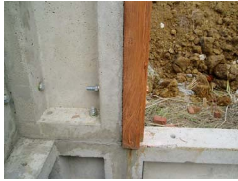
Figure 7. Pre-cast construction using 2 bolts for connections between components
