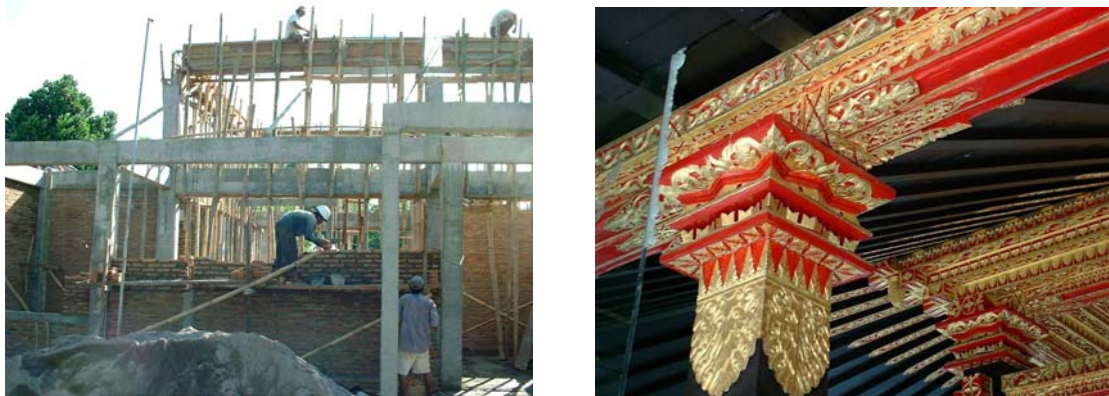
Figure 6. Recovery Works (Left) and the Traditional Construction of Java (Right), Yogyakarta, Indonesia, September 2006
