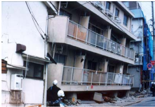
Figure 9. Soft first-story buildings (1995 Kobe Earthquake)
