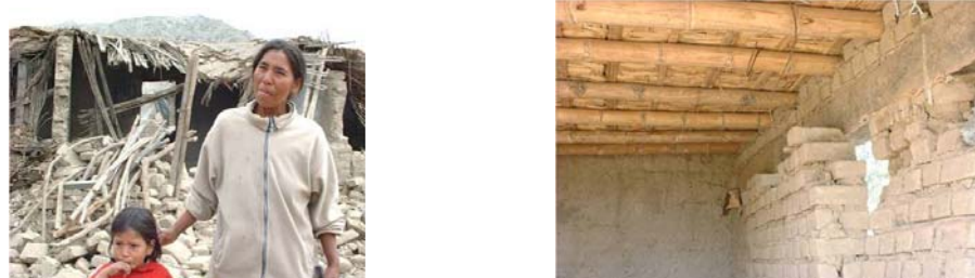
Figure 9. A Family Desperate after Losing their House by the 2007 Earthquake (Left) and Damage of Adobe-made House (Right), Pisco, Peru, August 2007
