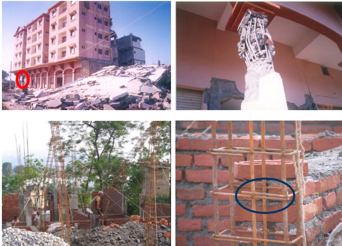
Figure 1. Collapse of a newly constructed building from 2001 Gujarat Earthquake (Left, top), improper detailing seen in one of the columns (Right, top) and a building under construction in Nepal (Bottom, left) where similar detailing is being practiced
