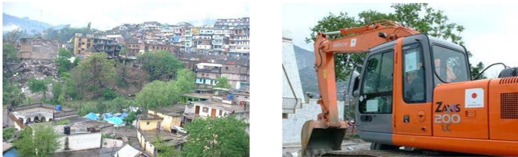
Figure 5. City of Muzaffarabad (Left) and the Operation of Reconstruction Works (Right), Muzaffarabad, Pakistan, March 2006
