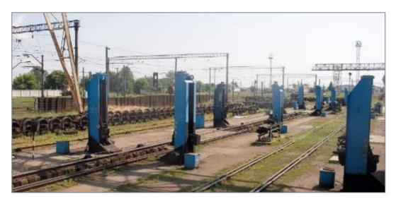
Figure 45: Bogie change station (Chop, Ukraine, between Russian gauge and standard gauge)
