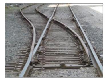
Figure 67: Switch and direction allowed
