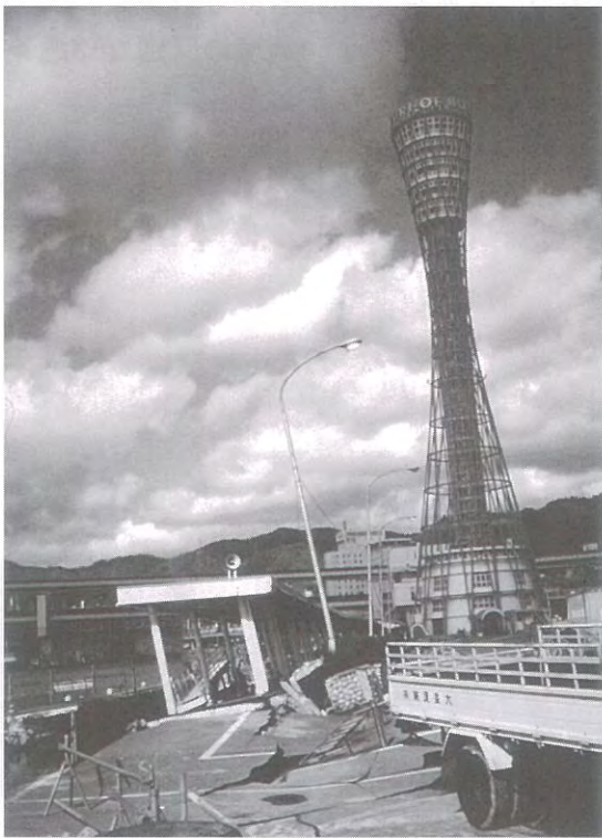
■ 1-1 Damage of the Kobe international port after the Great Hanshin-Awaji Earthquake reveals economic fragility of the port town.
