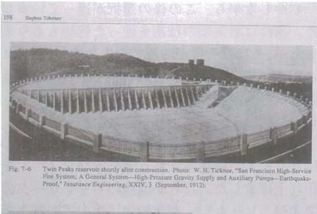
■ 1-25 Large reservoir tank in Twin Peaks, San Francisco. For the earthquake safety, the tank was divided into two areas.
