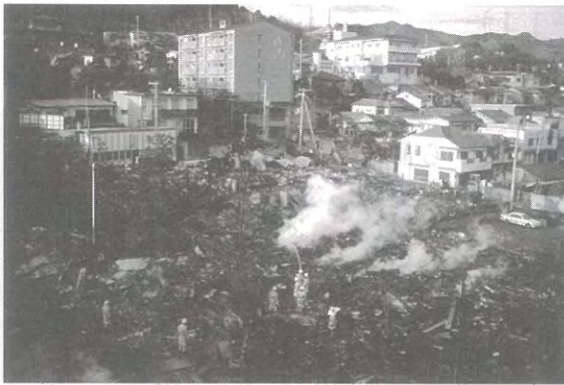
■ 1-7 The burned district. Several fire events broke out simultaneously after the shock, which was unexpected and far beyond the capacity to deal with.
