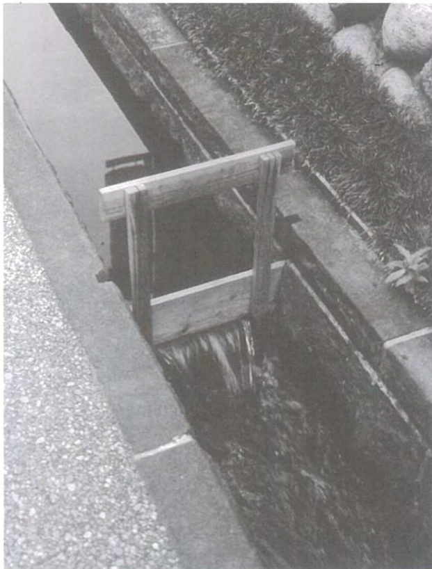
■ 1-59 Example of the adjustment system in the open stream.
