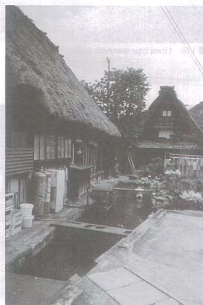
■ 1-48 Pond along each house was created in order to thaw the snow.
