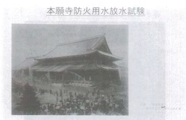
■ 1-75 Figure of the fire fighting drill using the water gun in Hongan-ji temple, Kyoto. This was a common practice in the past, but is not in use now.
