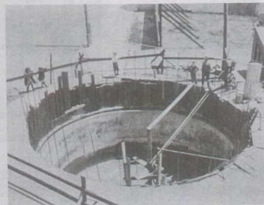
Fig. 7-16 Cisterns in construction in 1908. Photo: San Francisco Municipal Reports (1908-1909).
