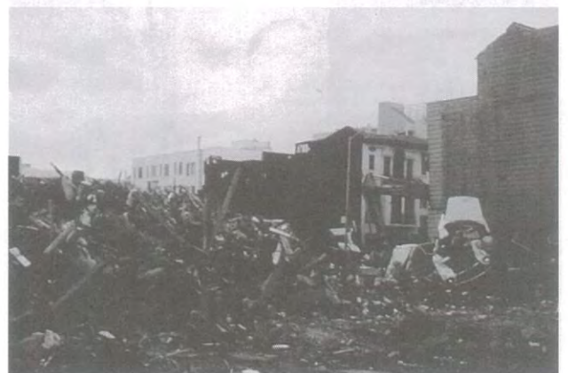
■ 1-36 Fire incident followed, but was prevented from spreading.
