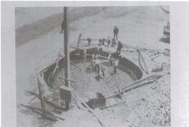
Fig. 7-15 Cisterns in construction in 1908. Photo: San Francisco Municipal Reports (1908-1909).
