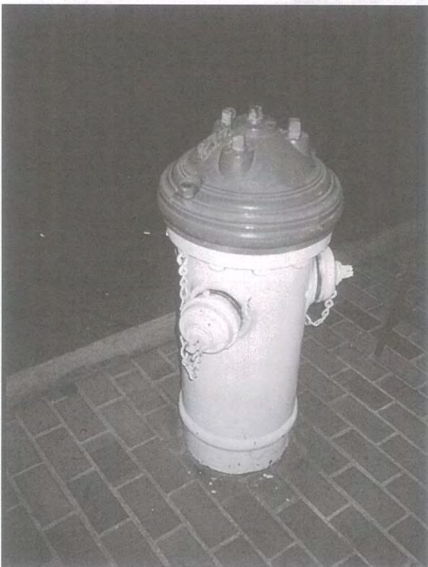
■ 1-30 Blue cap, a fireplug located on the lower zone. (S.F.)
