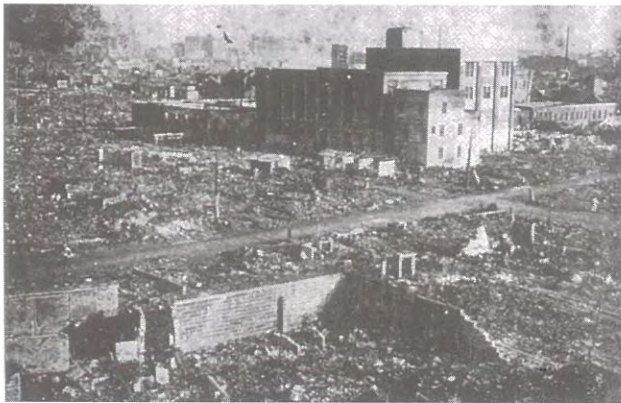
■ 1-12 Widely spread fire burning down several wooden areas completely.
