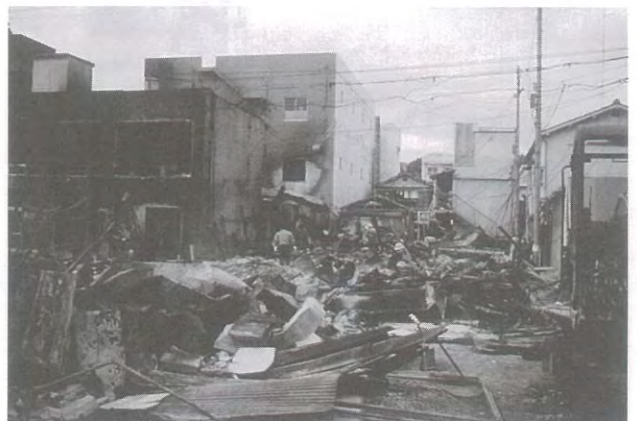
■ 1-6 Totally burned area. Many wooden buildings were suddenly collapsed, and then burned down after the disaster.
