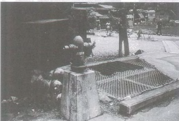
■ 1-51 Burial type reservoir tank.
