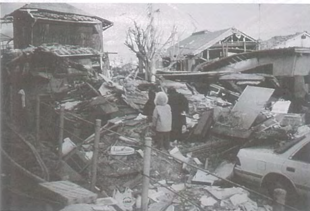
■ 1-5 Many old wooden houses were totally collapsed.
