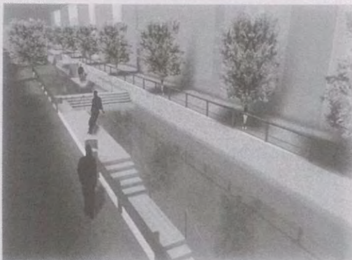
■ 1-71 Image of the reservoir system inside the stream using a series of dams.
