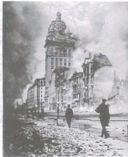
■ 1-20 Historical fire incident in San Francisco occurred after the earthquake in 1906.
