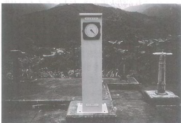
■ 1-45 Water pressure equipment.
