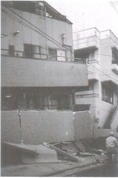
■ 1-3 Ground-floor parking lots were totally crushed particularly.
