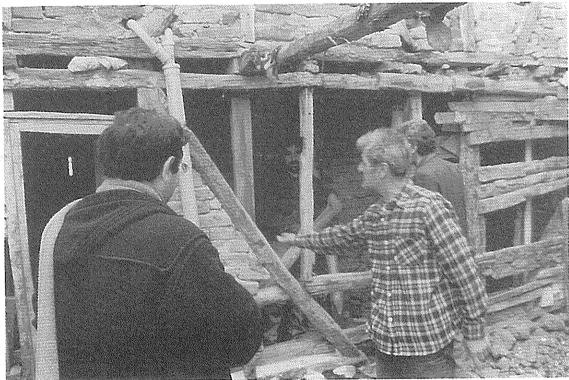
39. Derelict wooden building, İstanbul
