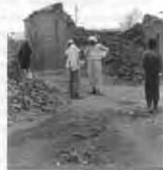
Damage in rural area
