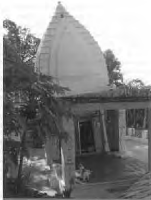
A temple affected in 1905 earthquake
