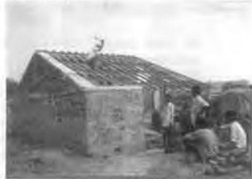
Construction of model house
