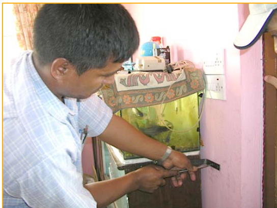
A trainer secures furniture using anchors in a community participant's home in Kathmandu.
