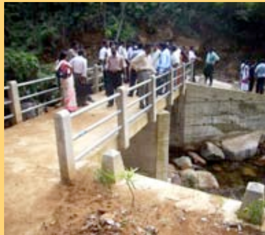
Field trip to observe the evacuation bridge.
