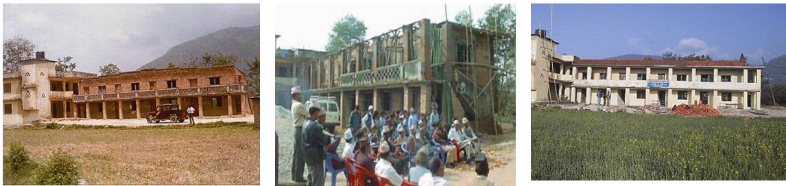
Figure 1.5 School Retrofitting in Nepal (2002): before - during - after (NSET) Discussion and observation of work were carried out during retrofitting.
