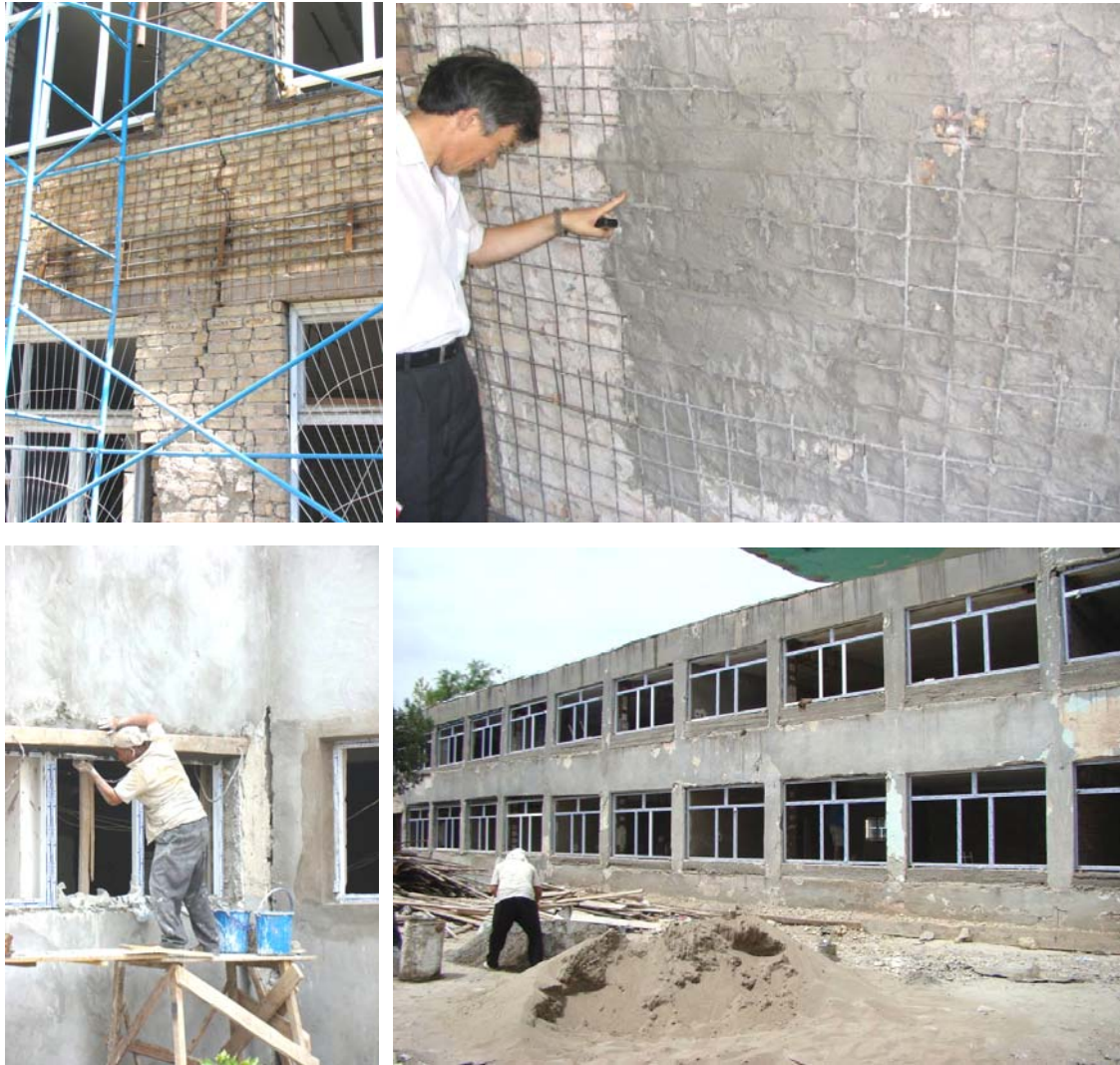
Figure 4.16: School building during retrofitting (Tashkent)
