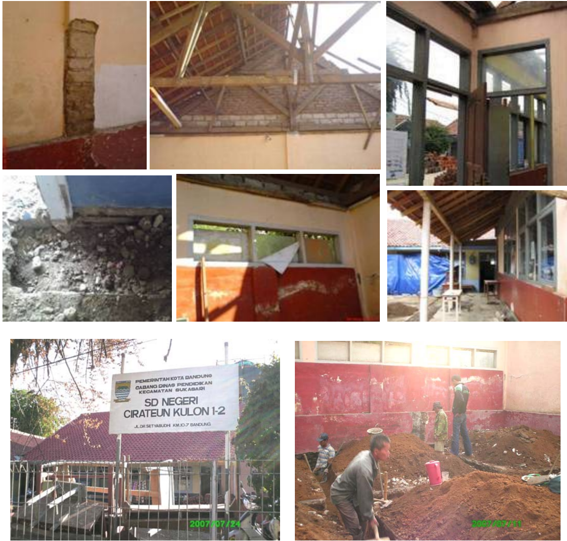
Figure 4.10 Existing structural conditions
