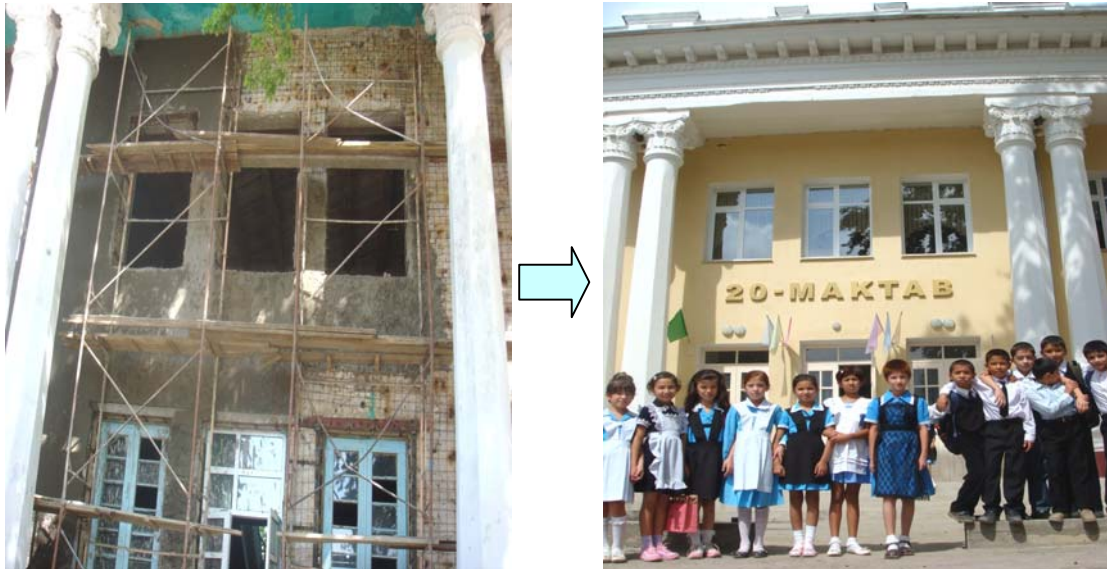
Figure 2.2 A School Building in Tashkent during and after retrofitting
