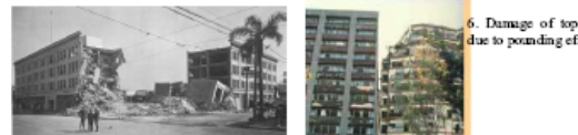
5. Collapse of an L-shaped Building 6. Damage of top floor due to pounding effect.
