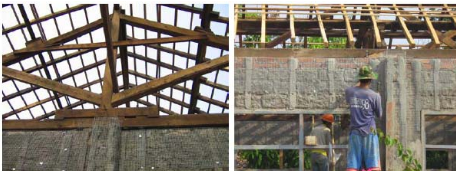
Figure 2.4 Retrofitting of a school in Indonesia
