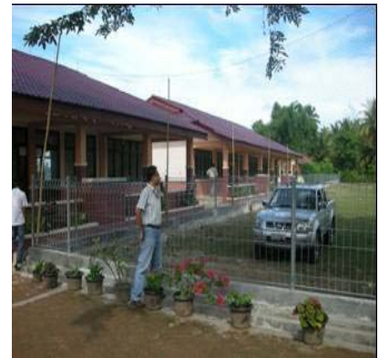
3: Retrofitted school building
