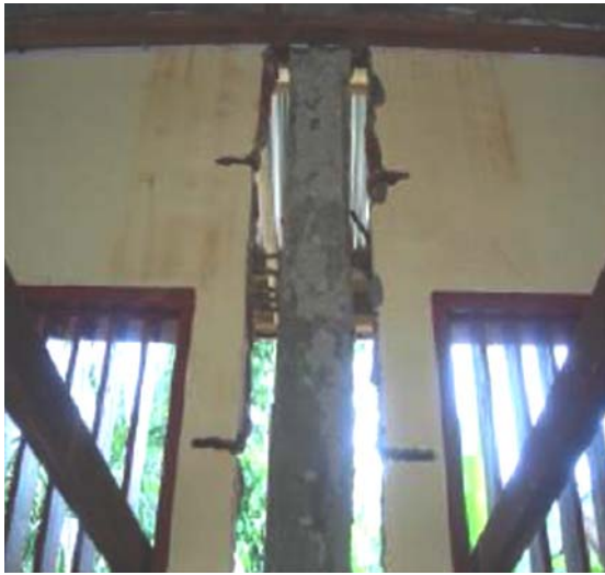
Column reinforcement and hook for connection to wall
