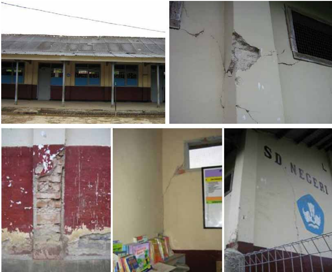
Figure 83: Existing condition of SD Padasuka II
