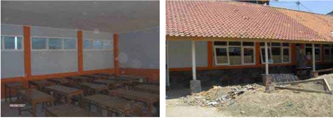
Figure 87: Various stages of the retrofitting process
