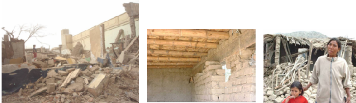
Figure: A Family Desperate after Losing their House by the 2007 Earthquake (Left) and Damage of Adobe-made House (Right), Pisco, Peru
