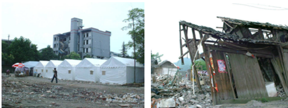
Figure: Temporary Shelters in Dujiangyuan (Left) Damage on Traditional Construction (Right), and Traditional Construction in the Region (Bottom), Sichuan Province, China, Aug 2008
