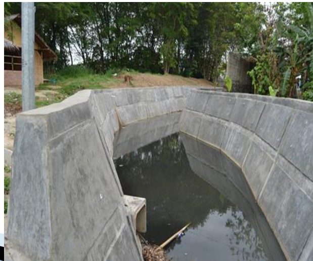
Embankment & Plaster Construction
