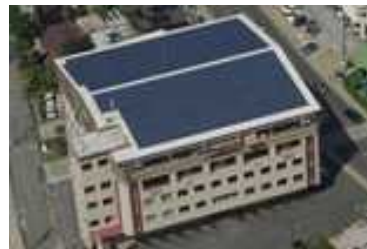
Installing solar PV system, PCKK, Palau Maldives
