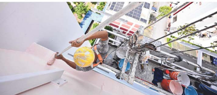
▲ A worker using cool paint, which can reduce surface heat absorption and emission, to paint the external walls of Block 848 Tampines Street 82 on Feb 3.
