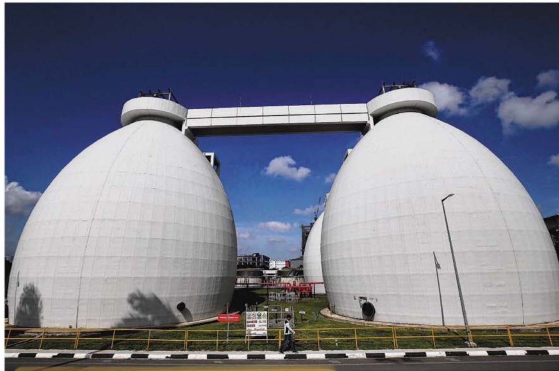
Sludge from the used water treatment process is converted to biogas in egg-shaped digesters at the Jurong Water Reclamation Plant. A major source of water demand growth is expected to be the non-domestic sector, where it is projected to increase from 55 per cent of total consumption now to over 60 per cent. ST FILE PHOTO
