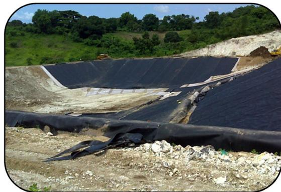
Photo 2 A cell of the landfill is being covered with clay and geosynthetic liner system during its construction.
