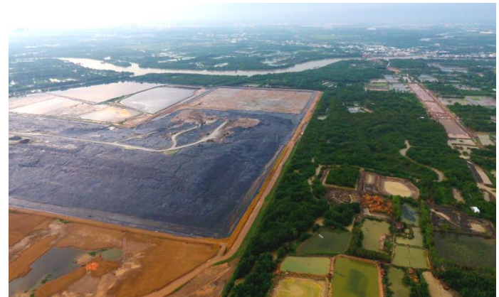
Da Phuoc landfill (Ho Chi Minh City) caused bad smelt to residential area
