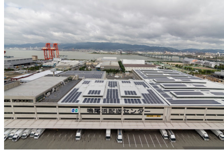
Naruohama Solar Power Plant
